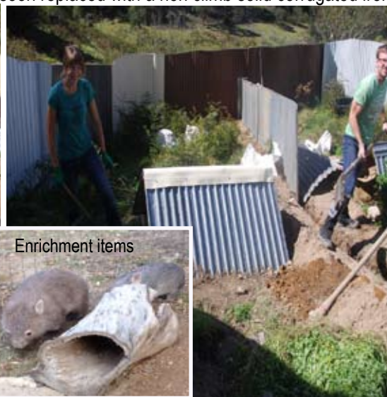
The temporary mesh divider was soon replaced with a non climb solid corrugated iron internal wall.
