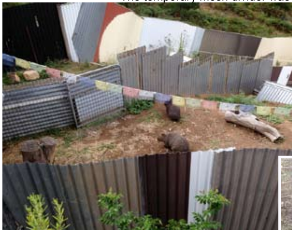
The temporary mesh divider was soon replaced with a non climb solid corrugated iron internal wall.
